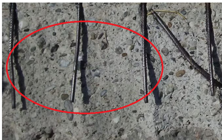
Fig.3.1 – Armature in alveo abrase.
